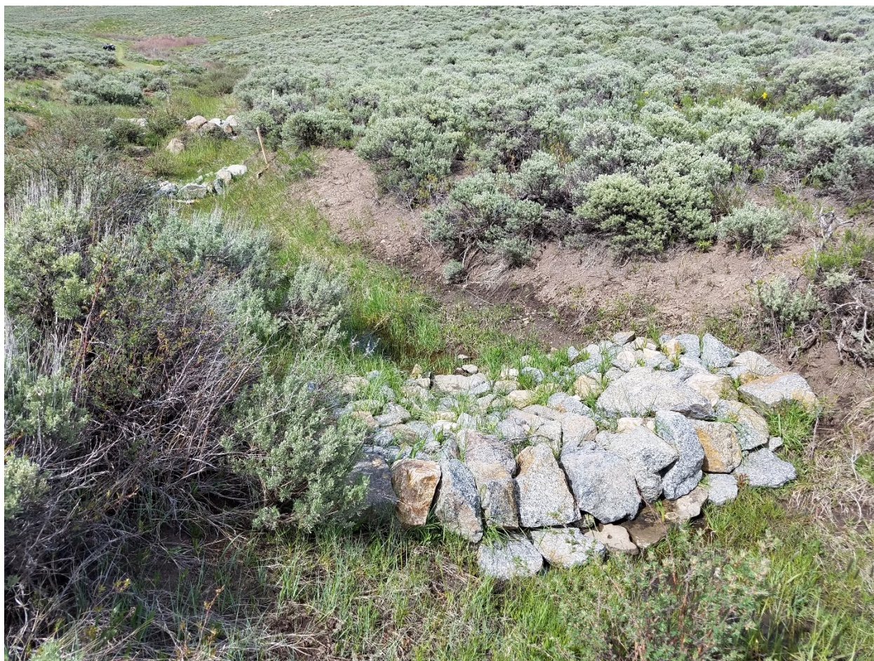
Zeedyk rock structures installed to restore incised channel. Photo by: Nathan Seward
