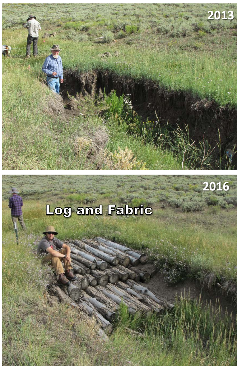
Figure 13. Log and fabric structure for treating headcuts before (top) and after (bottom) installation. Photos by: Renee Rondeau
