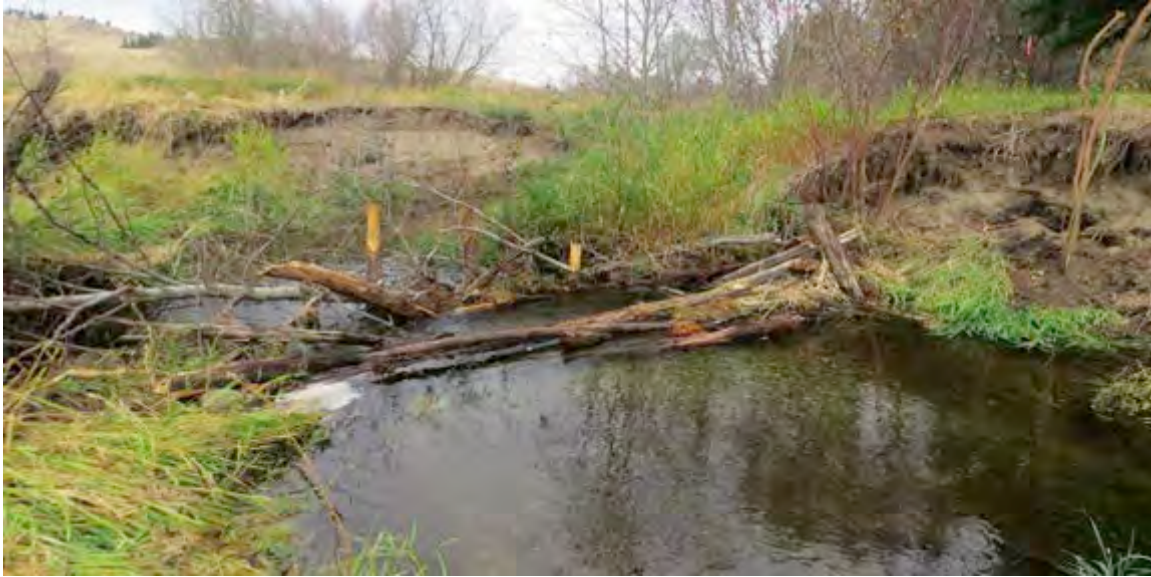
Figure 82: 12 days following installation of a BDA (same location as figure 81) and placement of LWD and other debris showing water pooling upstream
