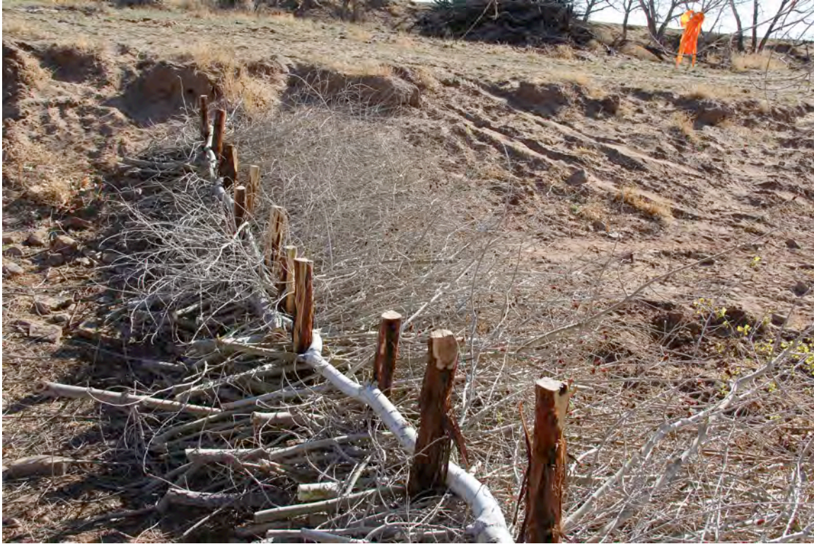
Figure 87: BDA interwoven with cottonwood branches parallel and perpendicular to the stream flow. The perpendicular, downstream (left to right) branches are placed to limit the development of a downstream scour pool during high-flow events, which could compromise the integrity of the structure. Photo courtesy of Seventh-Generation Institute.
