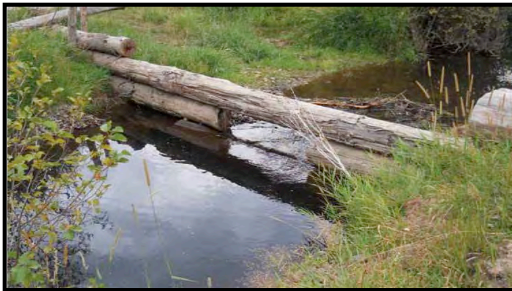
Figure 37: Flow-choke structures. These slow the movement of high-flow waters, increasing upstream flooding and creating temporary ponding, but during low flows they provide little functionality that is similar to a beaver dam. (From Devries et al. 2012).
