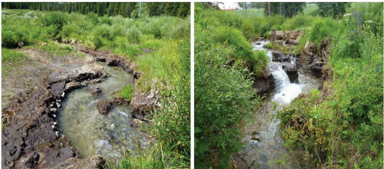
Figure 62: Once dams failed, a channel formed and immediately began head cutting. These photos show the Boreas Creek channel in different stages of incision, initial channel formation (left) and advanced incision (right)
