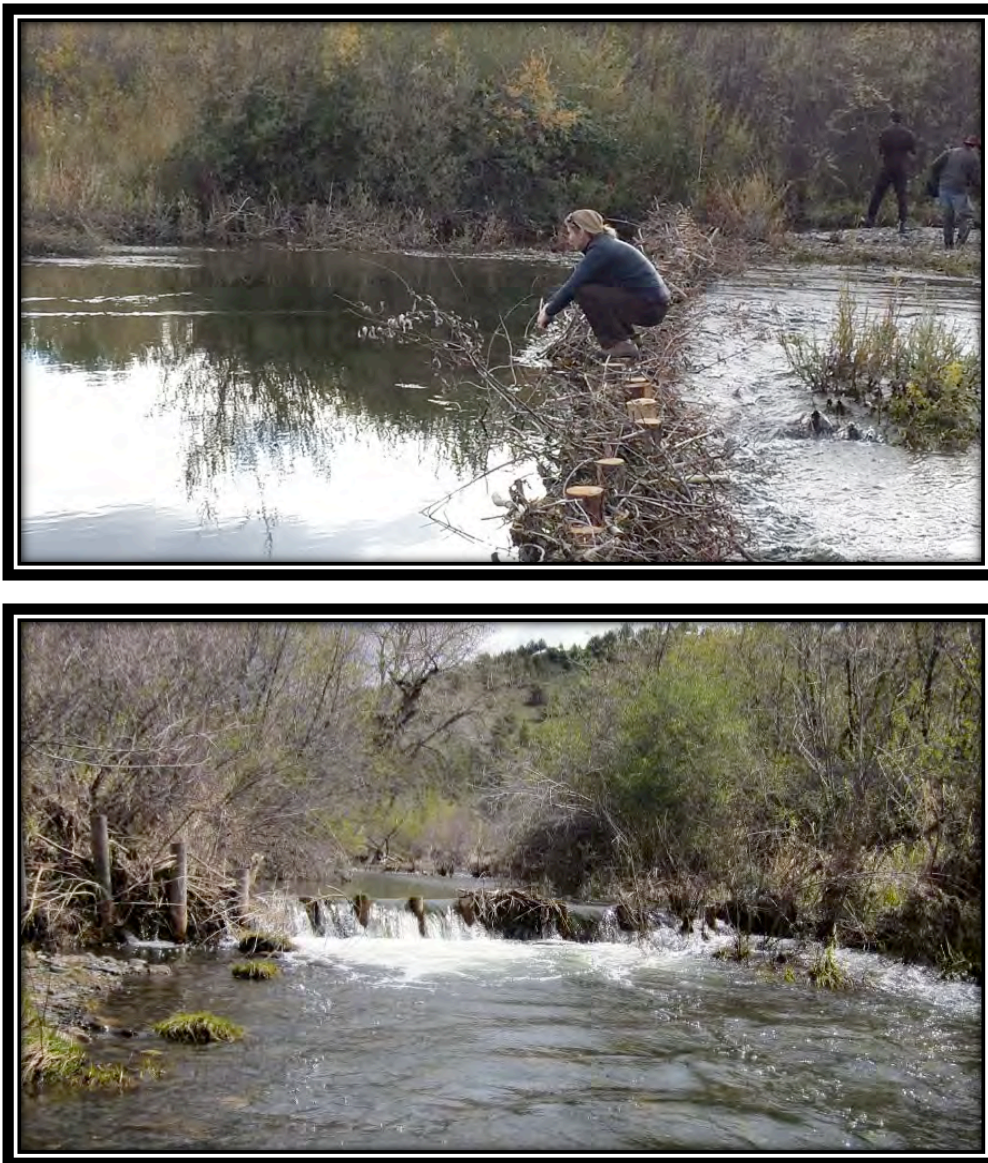
Figure 23: Examples of beaver dam analogues in Oregon and California.
